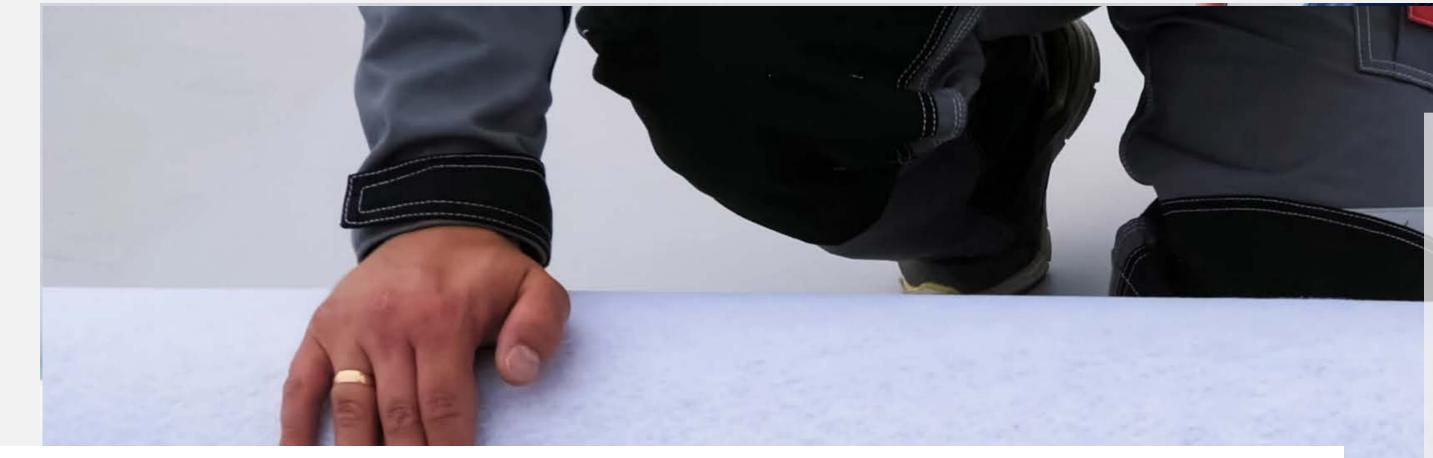
If you have a low-slope roof (also commonly called a flat roof, although this isn't strictly accurate), modified bitumen could be exactly the roofing material that you're looking for. Called "mod-bit" by roofers, this material is a membrane made of asphalt combined with polymerized rubber or plastic, and then it's further reinforced with fiberglass or another material.
